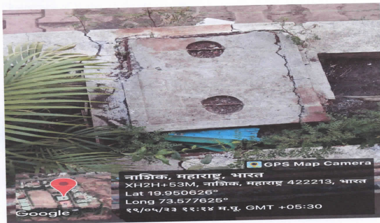
Photograph of Water Drainage Pit
