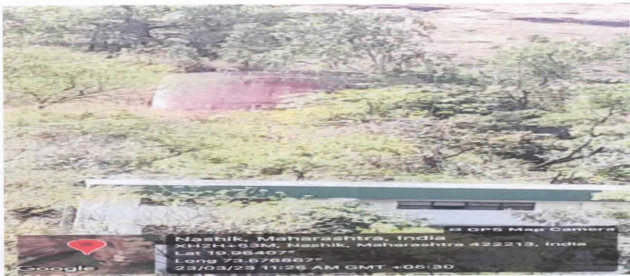
Photographs of Water Tank
