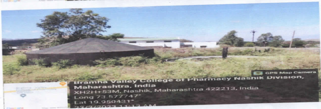
Photographs of Biogas Plant
